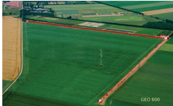
Figure 2.11: GEO600 land area, Sarsted, Germany (courtesy of GEO600 collaboration).
