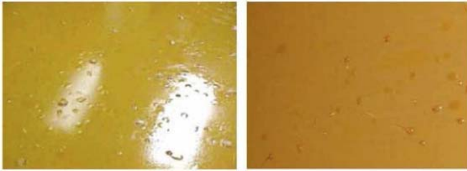
Figure 3.24: Photographs of defects on the linseed oil coating of a malfunctioning RPC.
