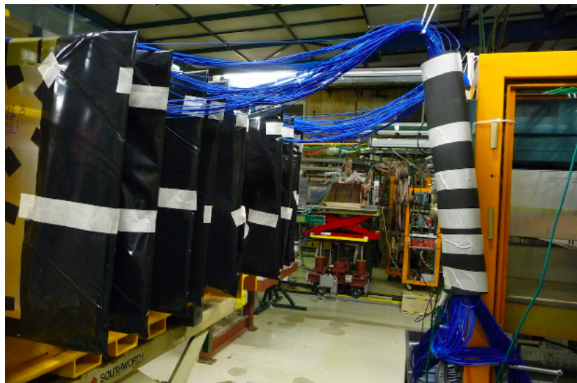
Figure 6.9: View of cabled layers.
