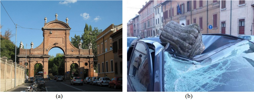
Fig.1 (a) Three-arched masonry city gate, Corso Giovecca, Ferrara, Italy; (b) damages from overturning of monolithic decorative elements during 2012 Emilia earthquake (Corso Giovecca, Ferrara, Italy).
