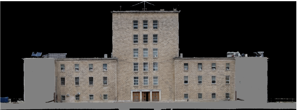
Figure 87. Image processed with photogrammeter of the facade from behind
