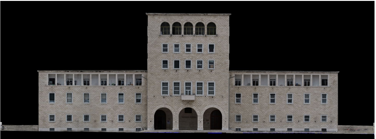
Figure 86. Image processed with photogrammetry of the main facade of the building
