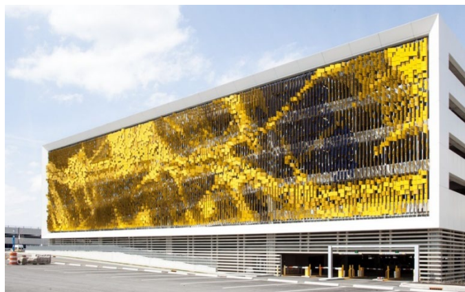
Fig. 4. Eskenazi Hospital parking structure, Rob Ley Studio (2014). Source: Rockinrollblues, CC BY-SA 4.0, via Wikimedia Commons
