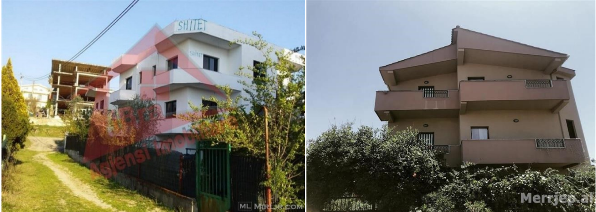
Figure 38: a) Private Villa in Durrës. Source: mirlir.com b) Private Villa in Golem. Source: merrjep.al
