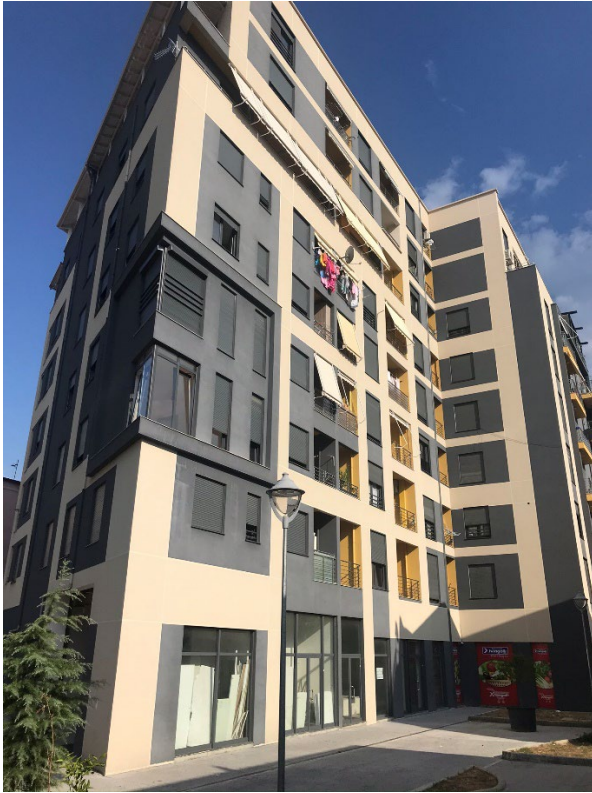
Figure 33: The palace built where there used to be a monument declared for preliminary protection with map code VI-35_zone CUS_5. Source: Author, 2020
