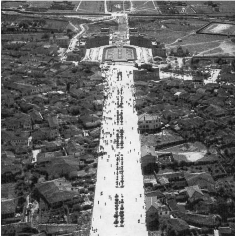
Figure 12: Air photo of the built Brassini Boulevard in the 30s Source: Archive of Polis University
