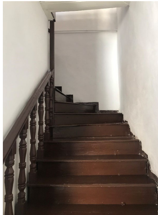
Figure 39: The interior stairs of the villa. Source:
