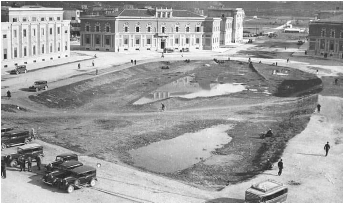
Figure 27: Skënderbej Square under construction. Source: Polis University Archive
