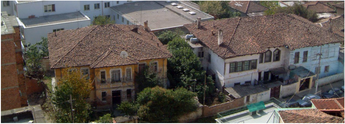
Figure 32: Toptanas villas aerial view in Tefta Tashko Street before the demolition; Source Citizen Channel
