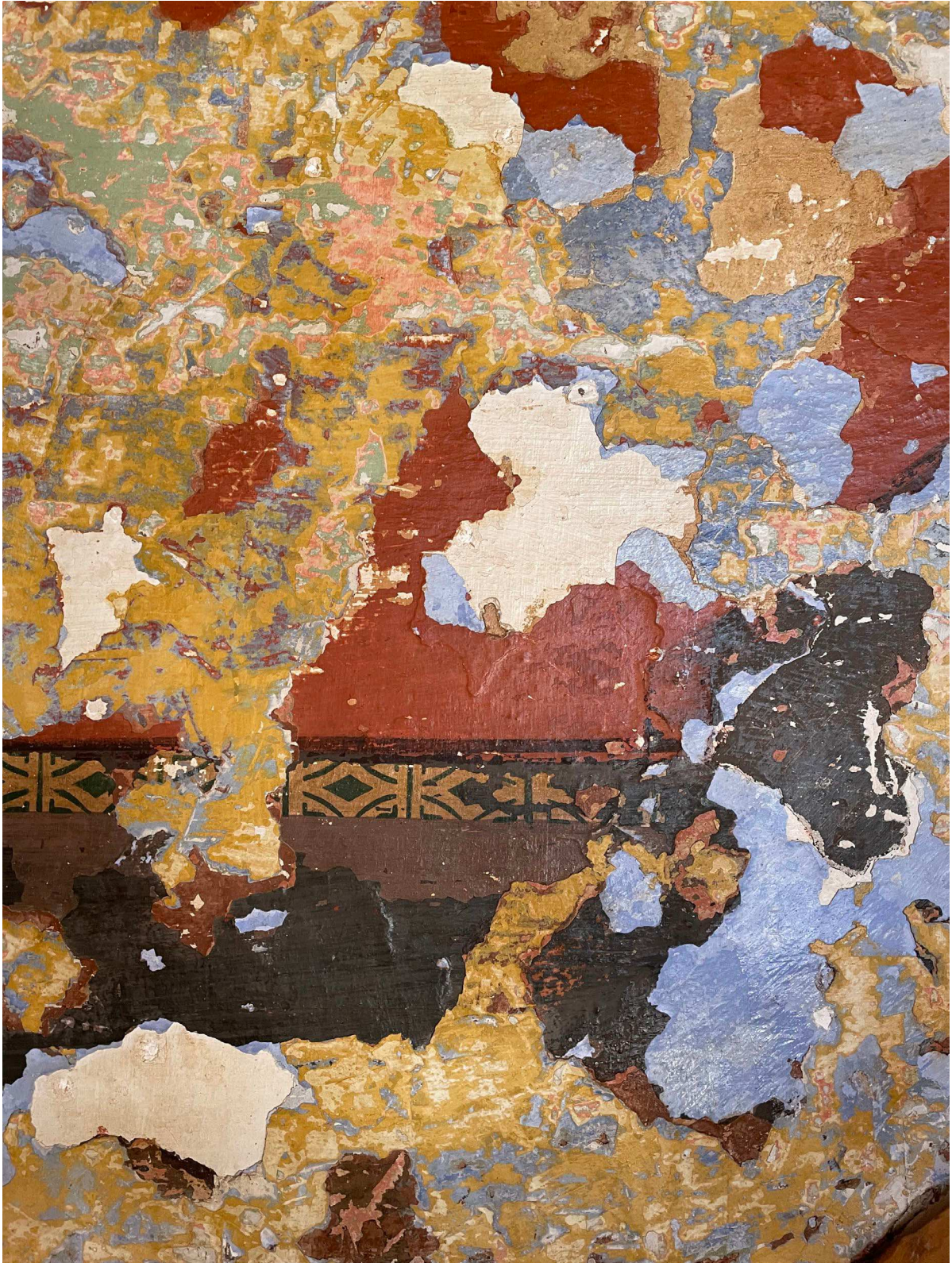
Wall color layers of a 19th-century house in the Old district of Tirana. Source: Author, 2022
