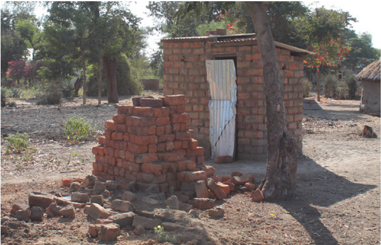
7.13 Traditional pit latrine in Maji Moto, close to a pile of fired bricks. Source: Own picture
