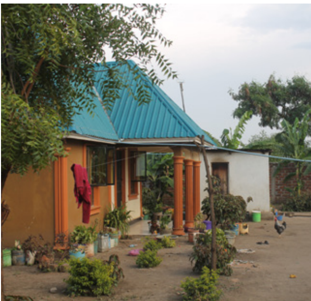
12.22 Flashy porch and entrance in Maji Moto, decorated with gypsum columns and well-maintained coloured plaster. Source: Own picture
