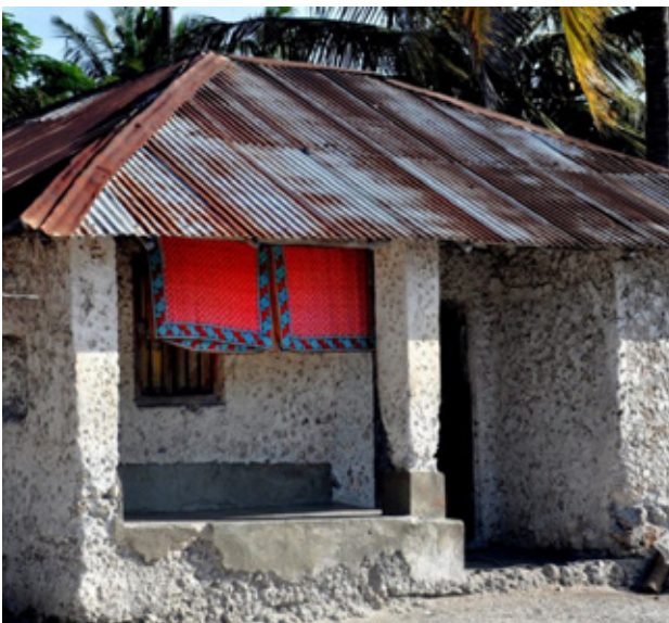
13.3 Traditional Swahili house with porch in Zanzibar. Source: Dominique Hazard
