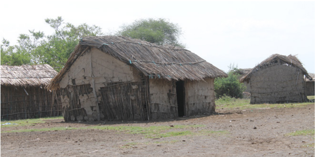
12.10 Due to the lack of continuous maintenance, mud houses built with the wattle and daub technique fall apart in Mikocheni. Source: Own picture
