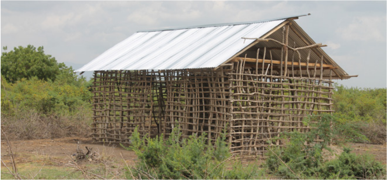
13.17 New house that Gabriel is building in a new by compound, built with wattle and daub but differently from the current one, roofed with CIS. Source: own picture
