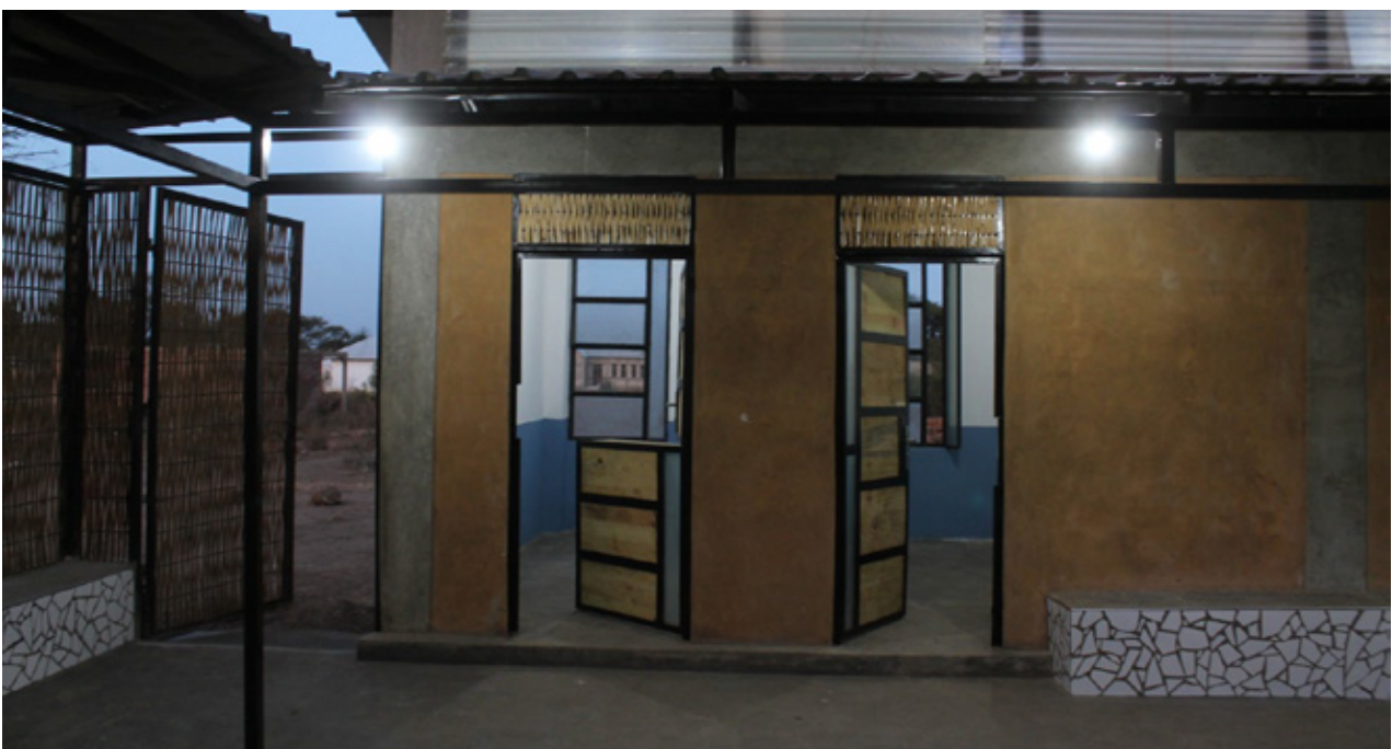
7.36 Night view of the reception room and open courtyard, with visible closing of the Vierendeel truss. Source: own picture
