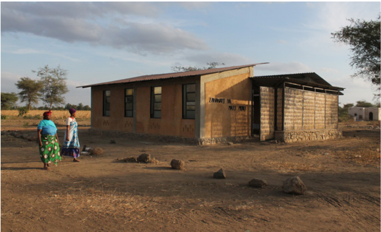
7.12 External view of the building, where the entrance and bamboo shading can be seen. Source: Own picture
