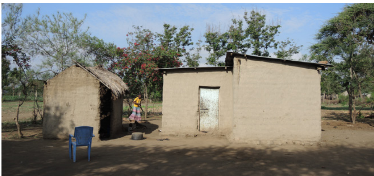
13.8 Family compound in Maji Moto with thatched building on the left used as kitchen and house roofed with CIS on the right, main house. Source: Own picture
