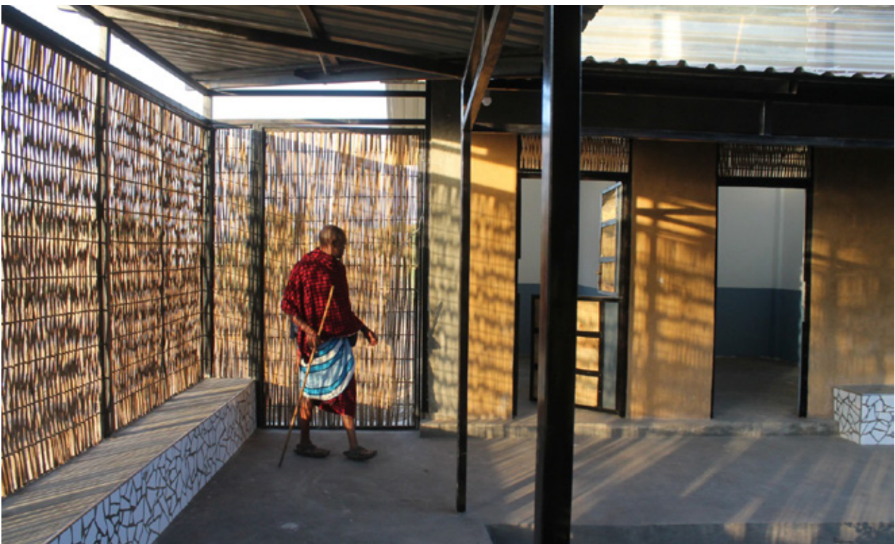
7.11 Dispensary's front wall, entrance and main courtyard, which highlights the bamboo lattice work. Source: Own picture
