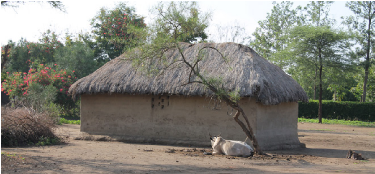
13.9 In traditionally built houses, windows are absent, with only some little openings to enable ventilation flow. Source: Own picture
