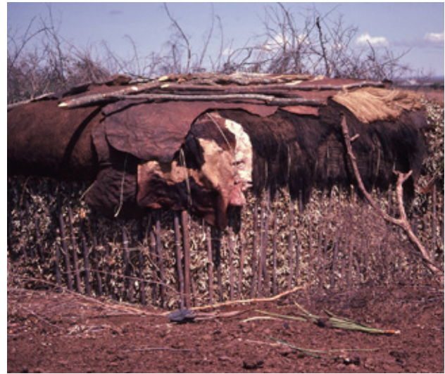
3.7 Enkaji covered with leather to avoid leaks during rainy season. Source: Jhon Tyman
