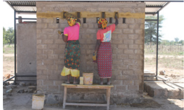
7.44 Women working on the colour plastering of the toilet block. Source: Own picture
