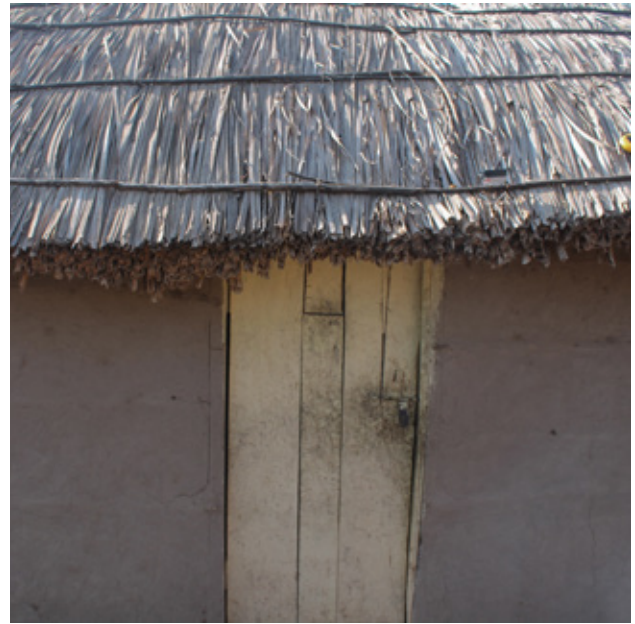
14.2 A thatched roof in a mud house in Mikocheni, denoting the thickness of the local reeds. Source: Own picture
