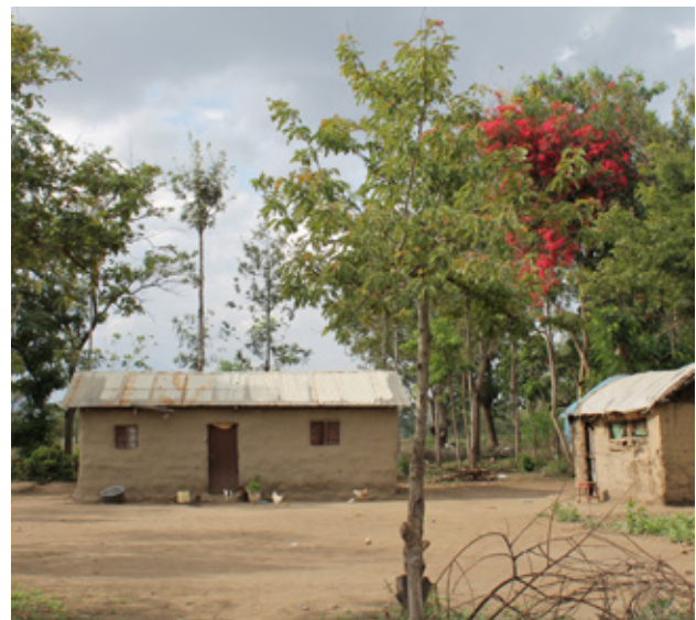
3.14 Boma in Maji Moto with two houses built with adobe bricks and plastered with mud. Source: Own picture
