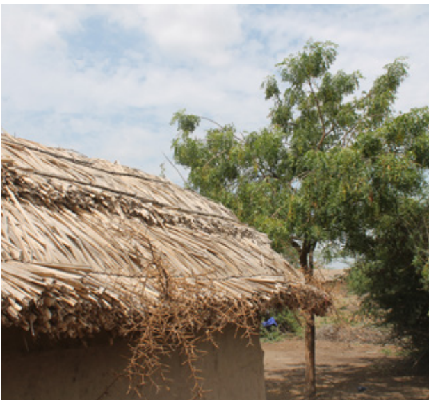
6.3 Thatched roof made from river reeds in Mikocheni. Source: Own picture
