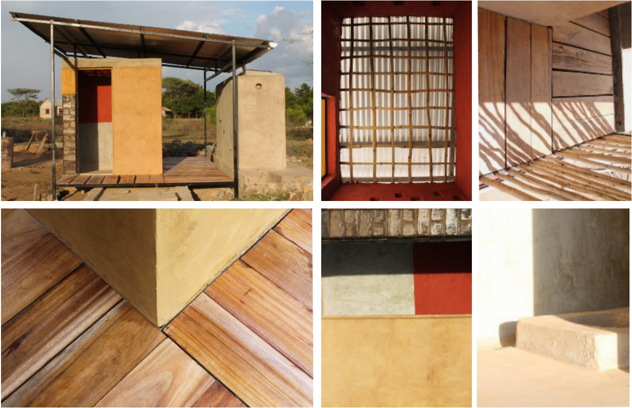
7.15 Details of the toilet block, wooden floor, bamboo mosquito net and paint. Source: Own picture
