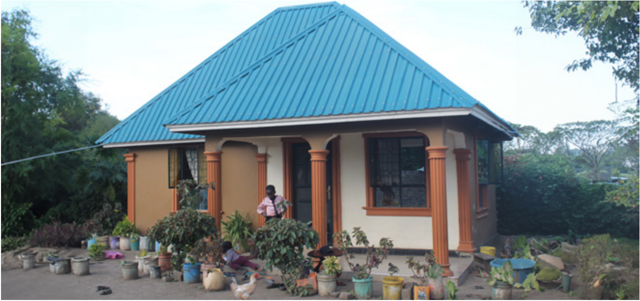
13.14 Front view of Balozi's house and floor plan in Maji Moto. Source: own picture
