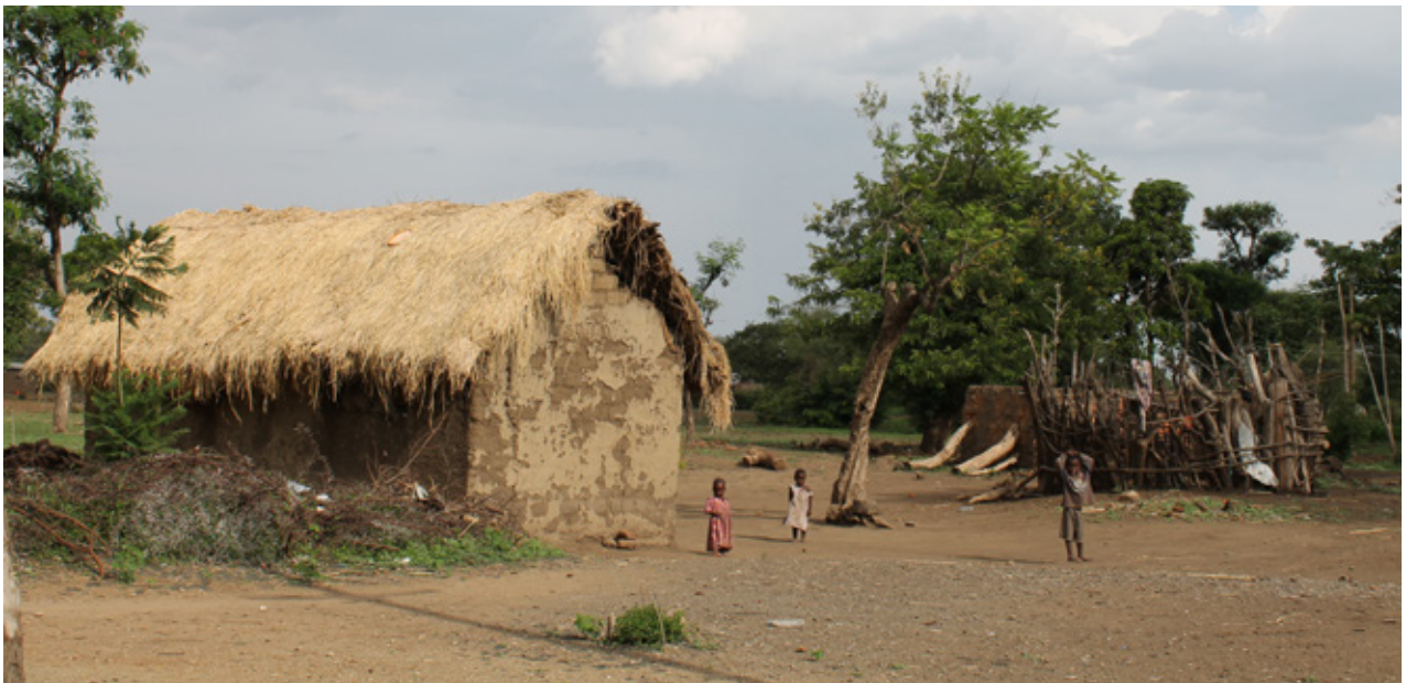
14.3 House built with adobe bricks and thatch in Maji Moto, which in this case is leftover straw. Note the difference of thatch in comparison to figure 14.2. Source: Own picture
