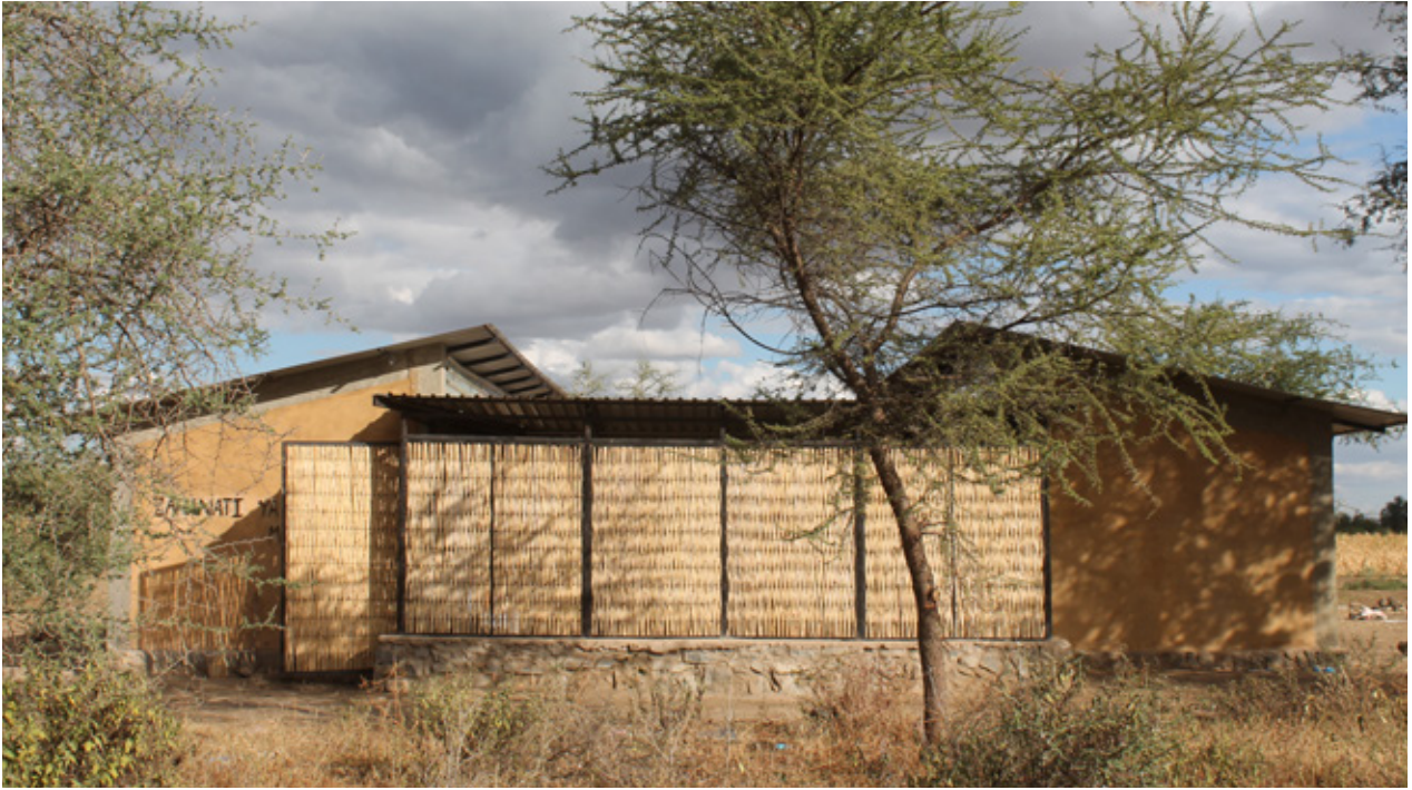
7.12 External view of the building, where the entrance and bamboo shading can be seen. Source: Own picture
