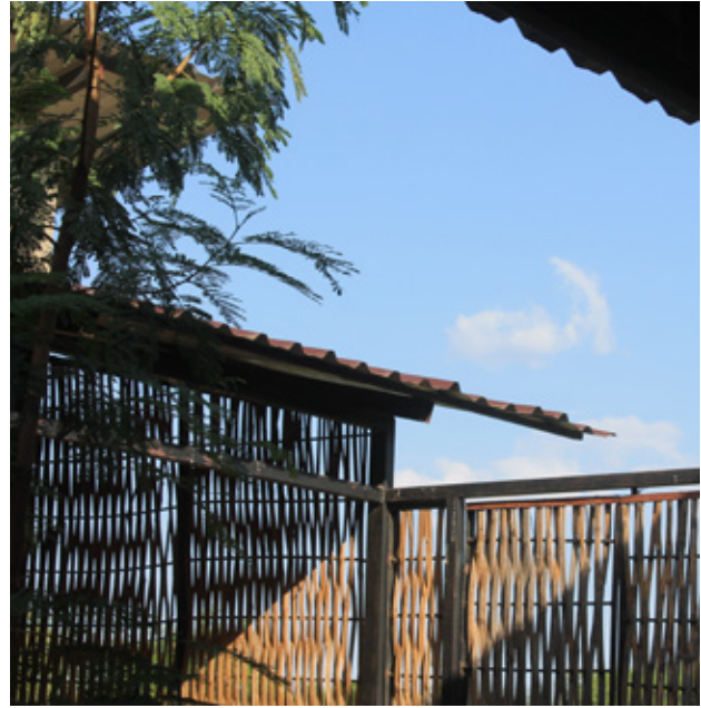
9.2 Steel structure for joining the bamboo lattice work on the back door. Source: Own picture
