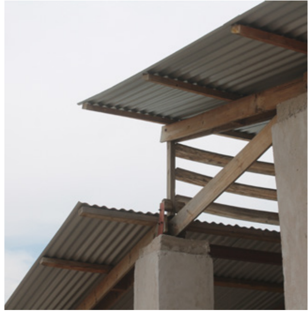
9.9 Detail of the open space created by the clerestory roof. Source: Own picture
