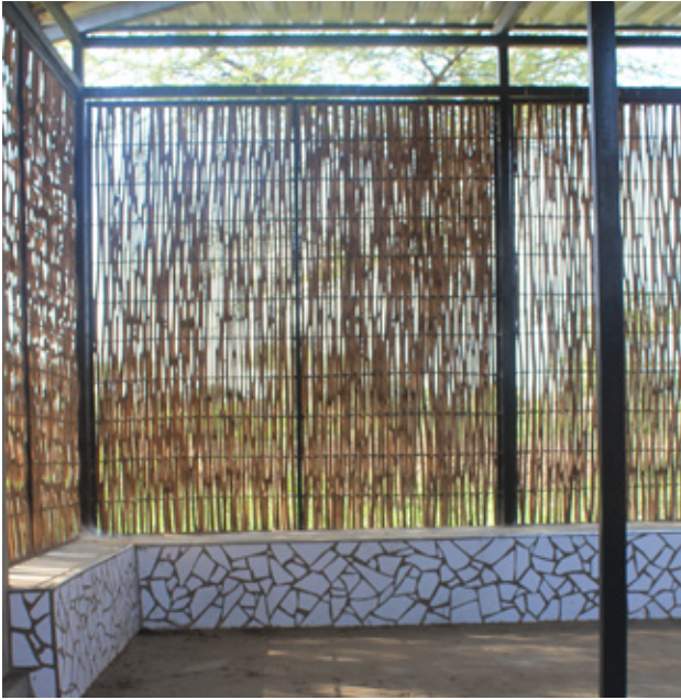
9.1 View of the health centre's waiting area, with tiled bench and its characteristic closing filter made with local bamboo. Source: Own picture
