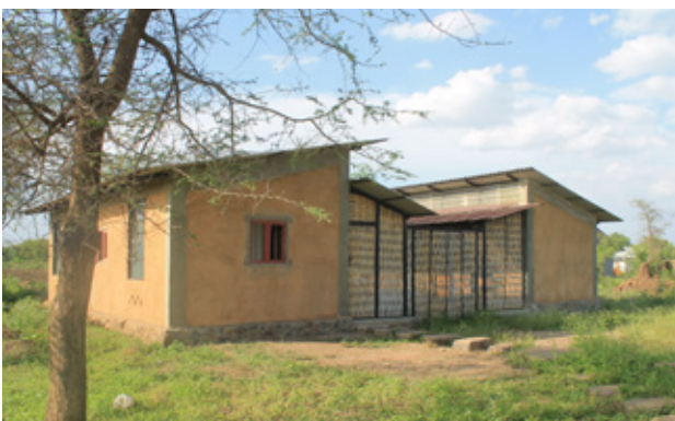
9.5 Back view of the health centre with the new additional window on the left-wing. Source: Own picture
