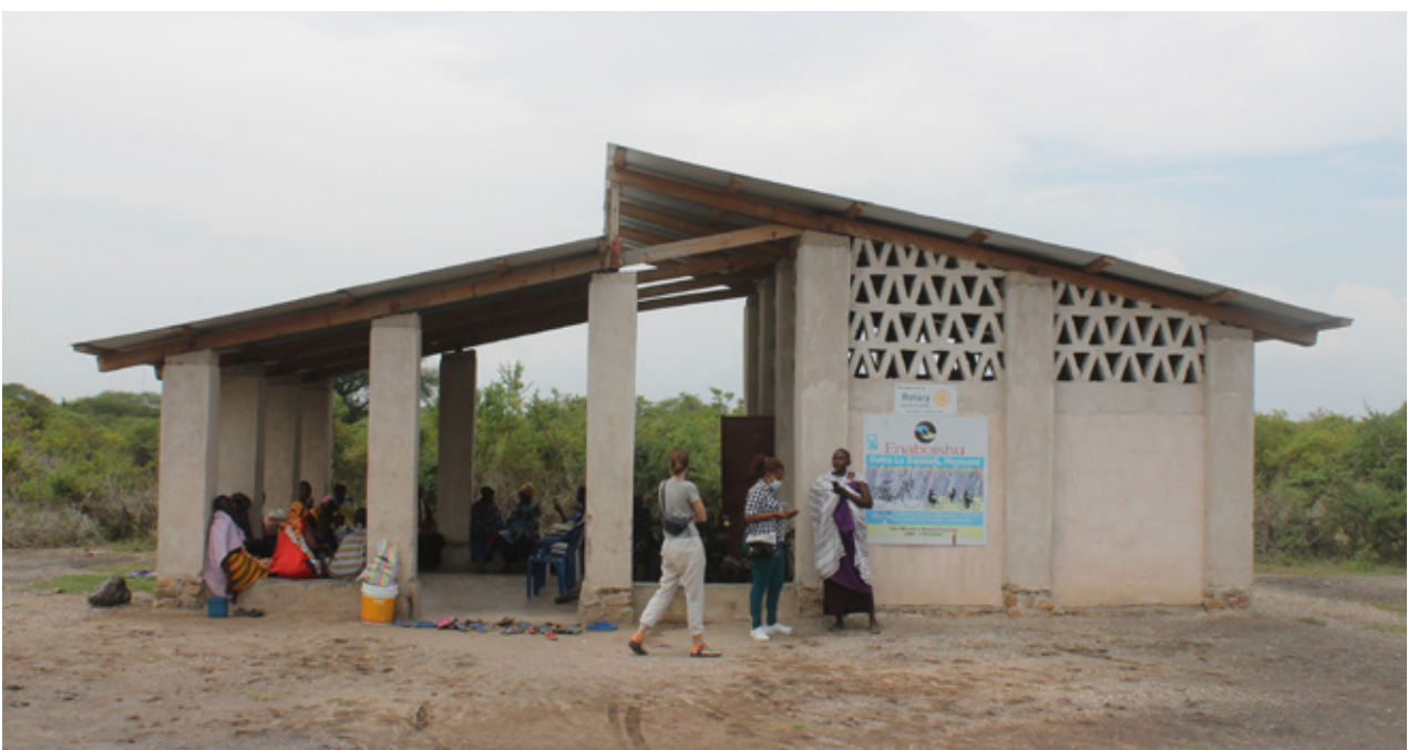
9.11 Front view of the bike shop where the newly plastered columns can be observed. Source: Own picture
