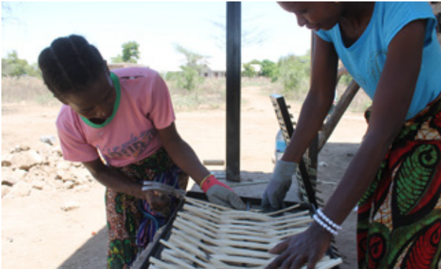
7.43 Women working on the construction of the bamboo windows. Source: Own picture
