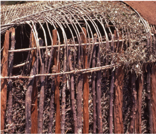
3.6 Maasai Enkaji under construction. Source: Jhon Tyman
