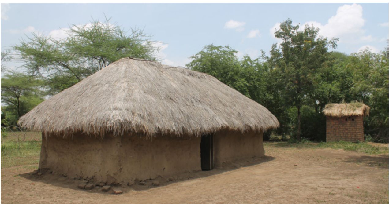
12.13 Moses's house side view and plan. To note the low height of the door and roof, due to the requirements of the thatch structure. Source: Own picture
