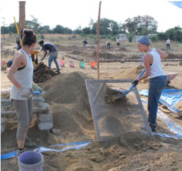
7.26 Volunteers sieving the excavated soil from the site before using it for producing the CSEB. Source: Own picture
