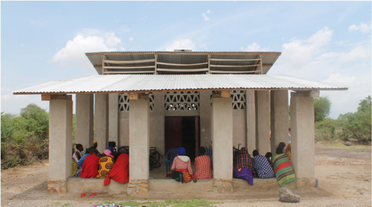
9.10 New look of the bike shop walls after the application of the cement plaster. Source: Own picture
