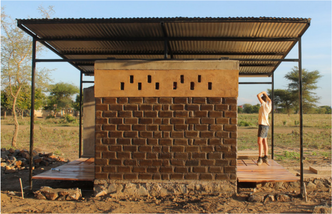
7.14 Dispensary's toilet block from the front and right side. See the water tank which collects rainwater. Source: Own picture
