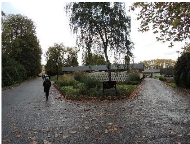
Figure 69 - The crematoria from the City of London Cemetery & Crematorium (London, UK) has solar panels installed on the rooftop, generating energy for the internal consumption of the cemetery.
