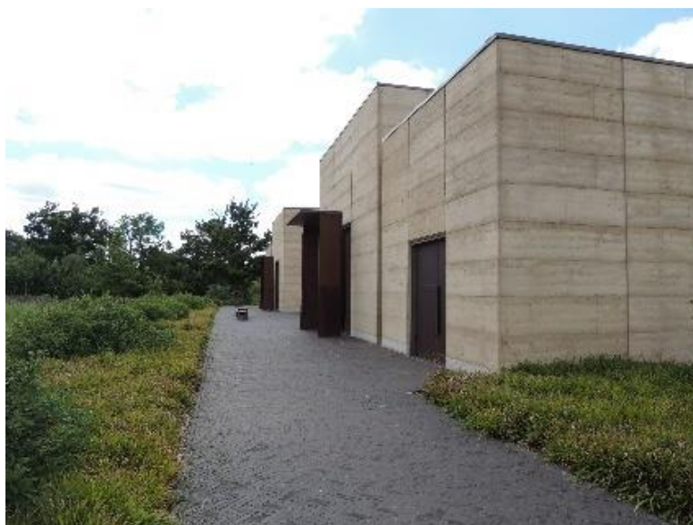
Figure 67 - Buildings from Bushey New Cemetery (London, UK) used for prayer halls and administrative offices and built with local sustainable materials.
