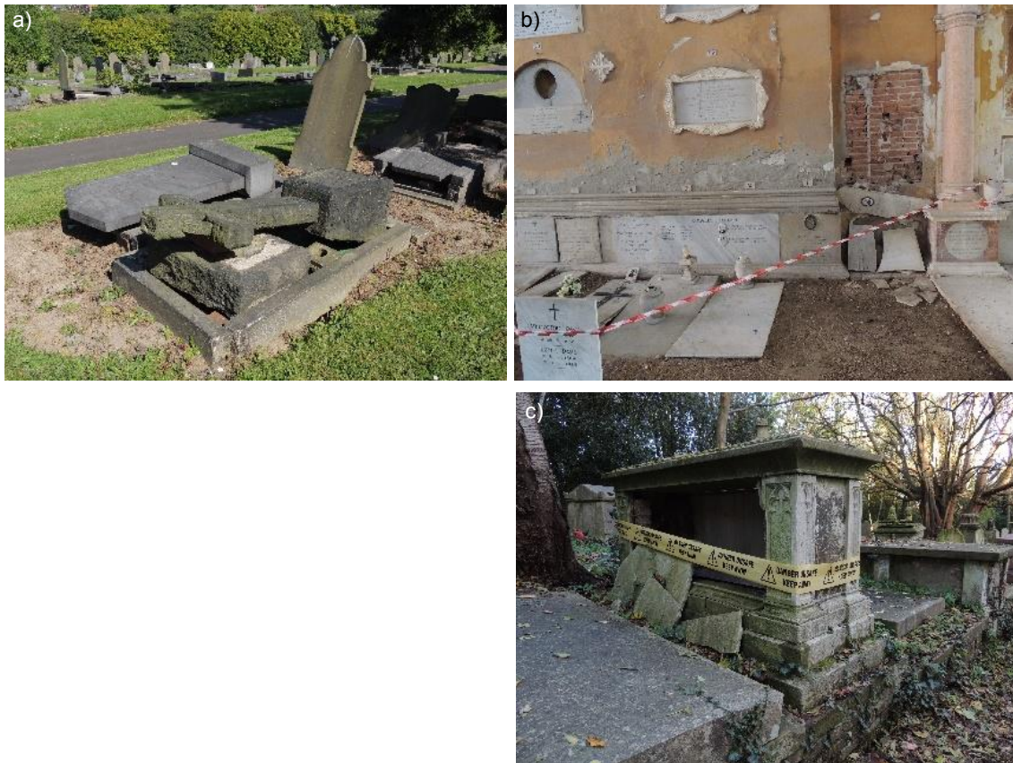
Figure 50 - Examples of risks for public safety: a) monuments laid down to avoid harming someone at the Abbey Lane Cemetery (Sheffield, UK); b) closed area for pedestrian access due to the risk of falling wall covering at the Cimitero Monumentale della Certosa di Ferrara (Ferrara, Italy); c) danger warning of monument instability at the Highgate Cemetery (London, UK).
