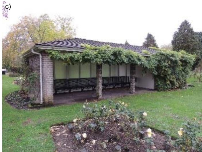
Figure 56 - Examples of unheated buildings and construction structures found at the site observation: a) toilets at the Bushey Old Cemetery (London, UK); b) religious sign at the Cemitério Municipal Água Verde (Curitiba, Brazil) 44 , where visitors can light candles instead of close to the burial space; c) sitting area within the City of London Cemetery & Crematorium (London, UK).
