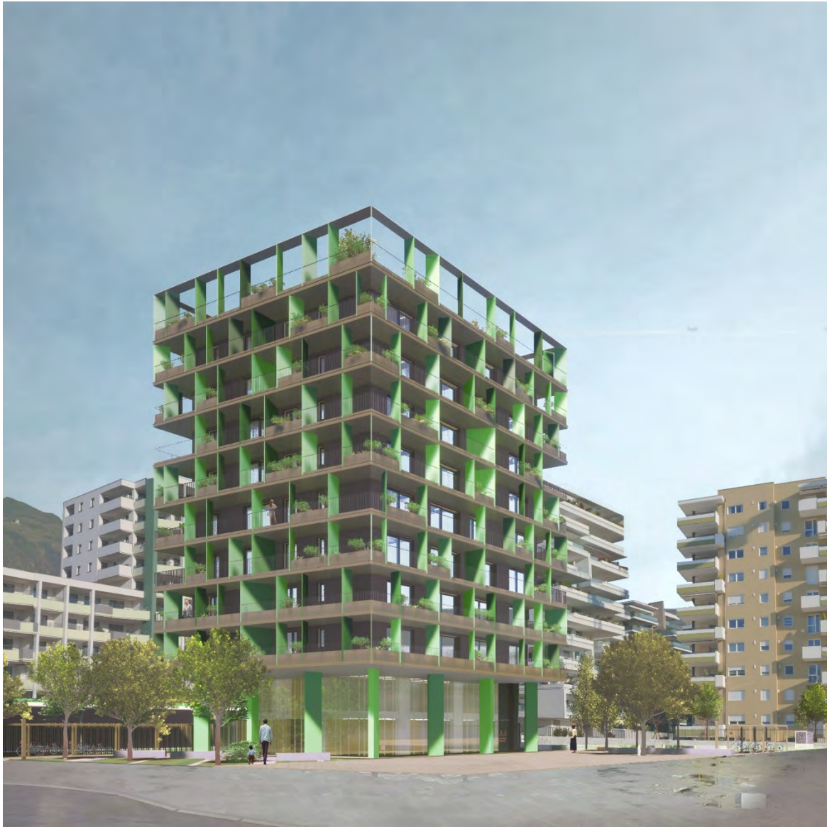
Figure 9. General view of building
