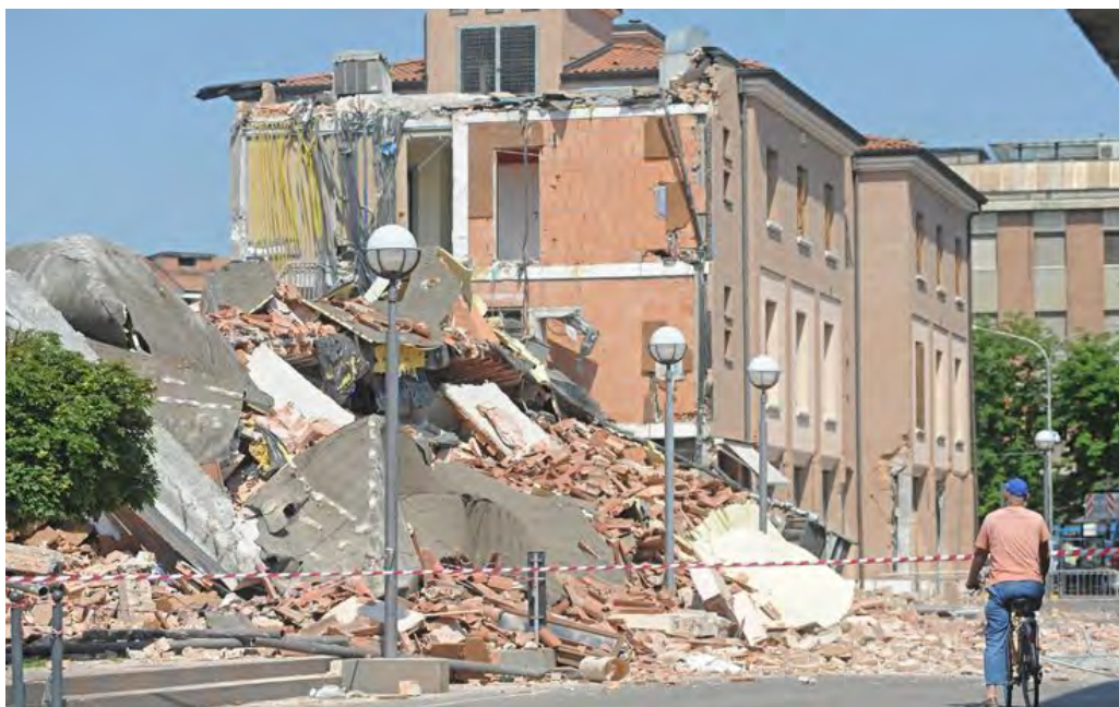
Figure 2. Residential building crashed in Cavezzo after the 2014 earthquake in Emilia Romagna land.
