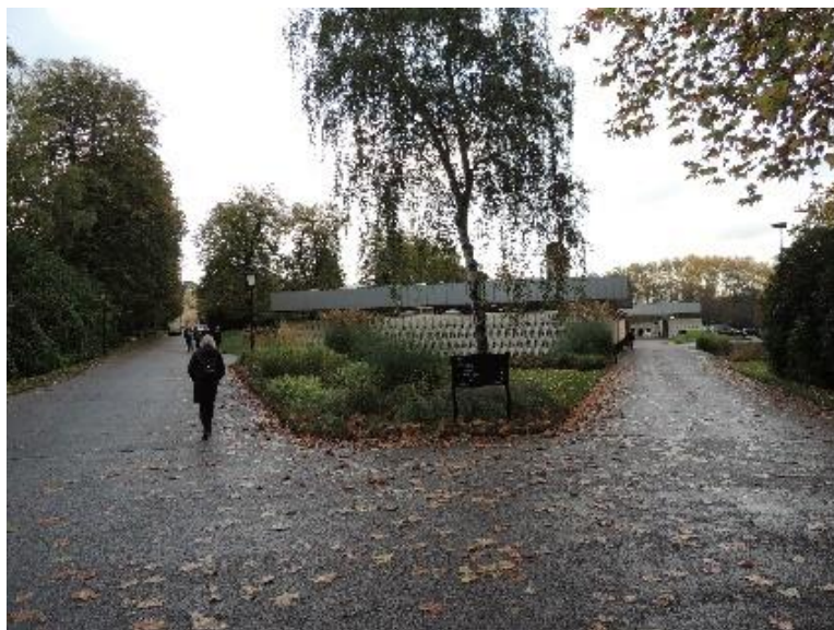
Figure 69 - The crematoria from the City of London Cemetery & Crematorium (London, UK) has solar panels installed on the rooftop, generating energy for the internal consumption of the cemetery.
