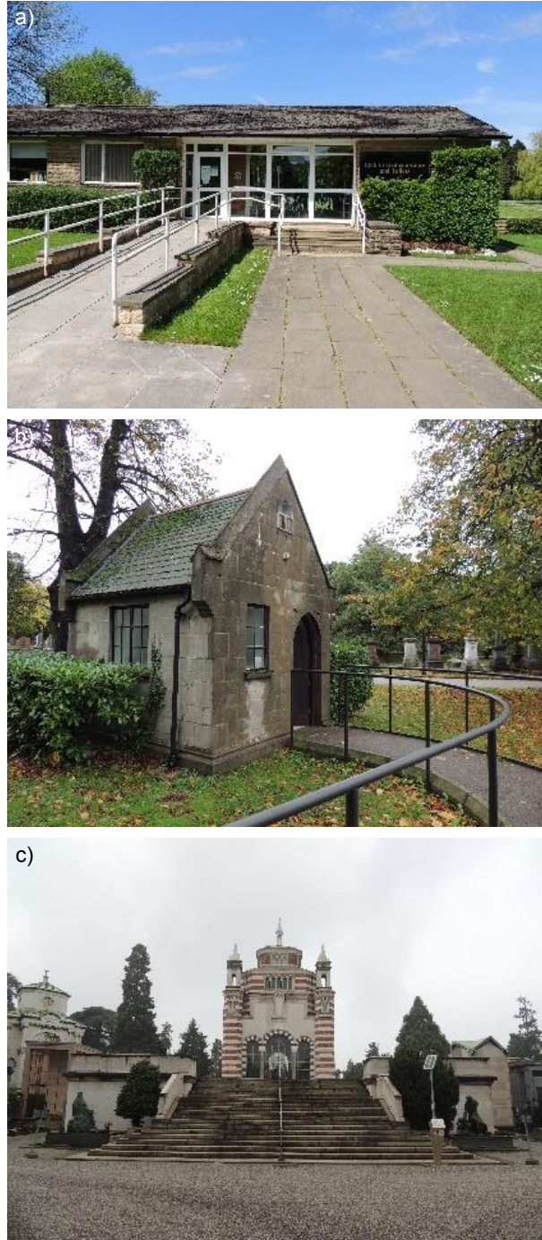
Figure 57 - Examples of accessible entrances: a) ramp and stairs of access at the Hall of Remembrance and Toilets at the Hutcliffe Wood Garden of Remembrance (Sheffield, UK); b) toilets and baby changing room fully equipped for disabled accessibility at the City of London Cemetery & Crematorium (London, UK); c) the historical character of the cemetery makes it difficult to install a disabled lift, leaving stairs as the only access the ossuary at the Cimitero Monumentale di Milano (Milan, Italy), but the handrail serves as a support for children, elderly any other person.
