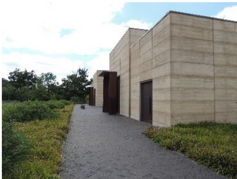
Figure 67 - Buildings from Bushey New Cemetery (London, UK) used for prayer halls and administrative offices and built with local sustainable materials.
