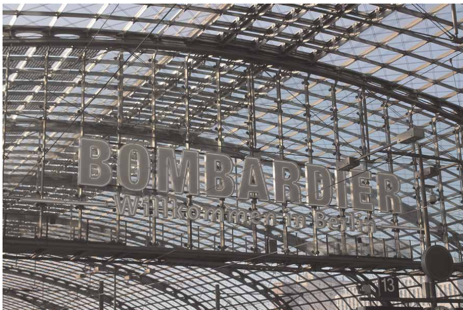
Figure 7. The Hauptbahnhof, Berlin (Germany): Detail of the 1700 m 2 curved surface covered with 780 semi-transparent c-Si panels (Energy output: 180 kWp, Architect: Meinhard von Gerkan; System provider: Optisol, 2003).
