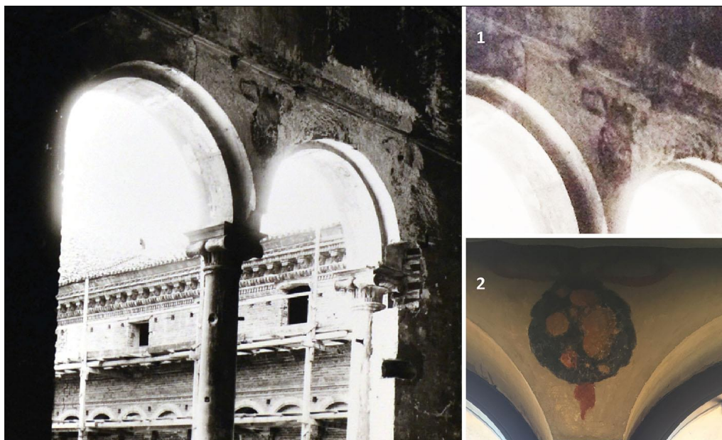
Figure 18. A Historical Photograph that Shows the Decorations Removed by the Restorations (1); These Decorations Were Identical to Those of the Pentafora as the Image on the Right Testifies (2)
