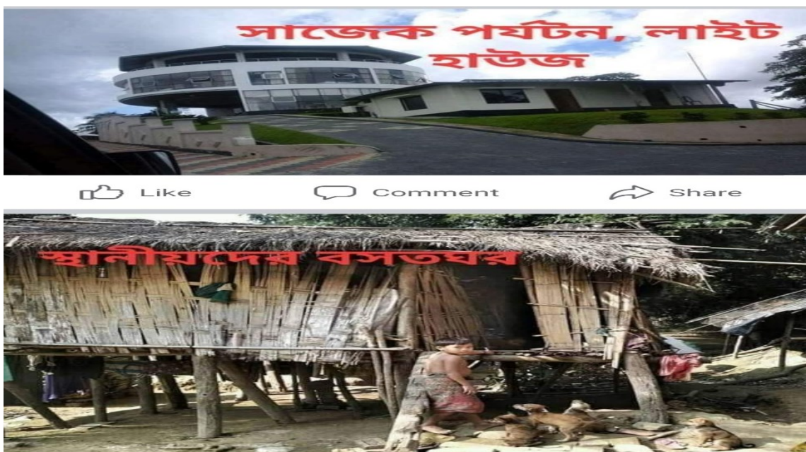
Figure-30: Luxury hotels for tourists, and dilapidated houses of locals. Source: Facebook (Our Khagrachari)
