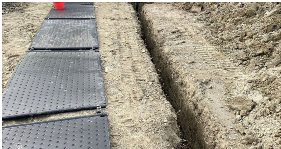
Fig. 1 Flat-panel GHE and trench for the installation
