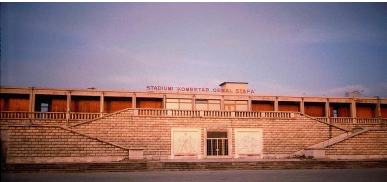
Figure 17: Entrance of the Air Albania national Stadium
