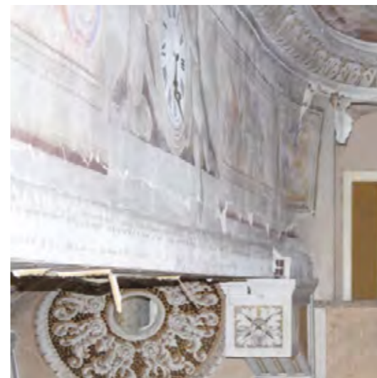
Detail views showing beam and scenic arch injuries
