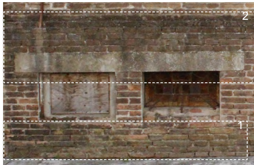
photographic survey_ north elevation
