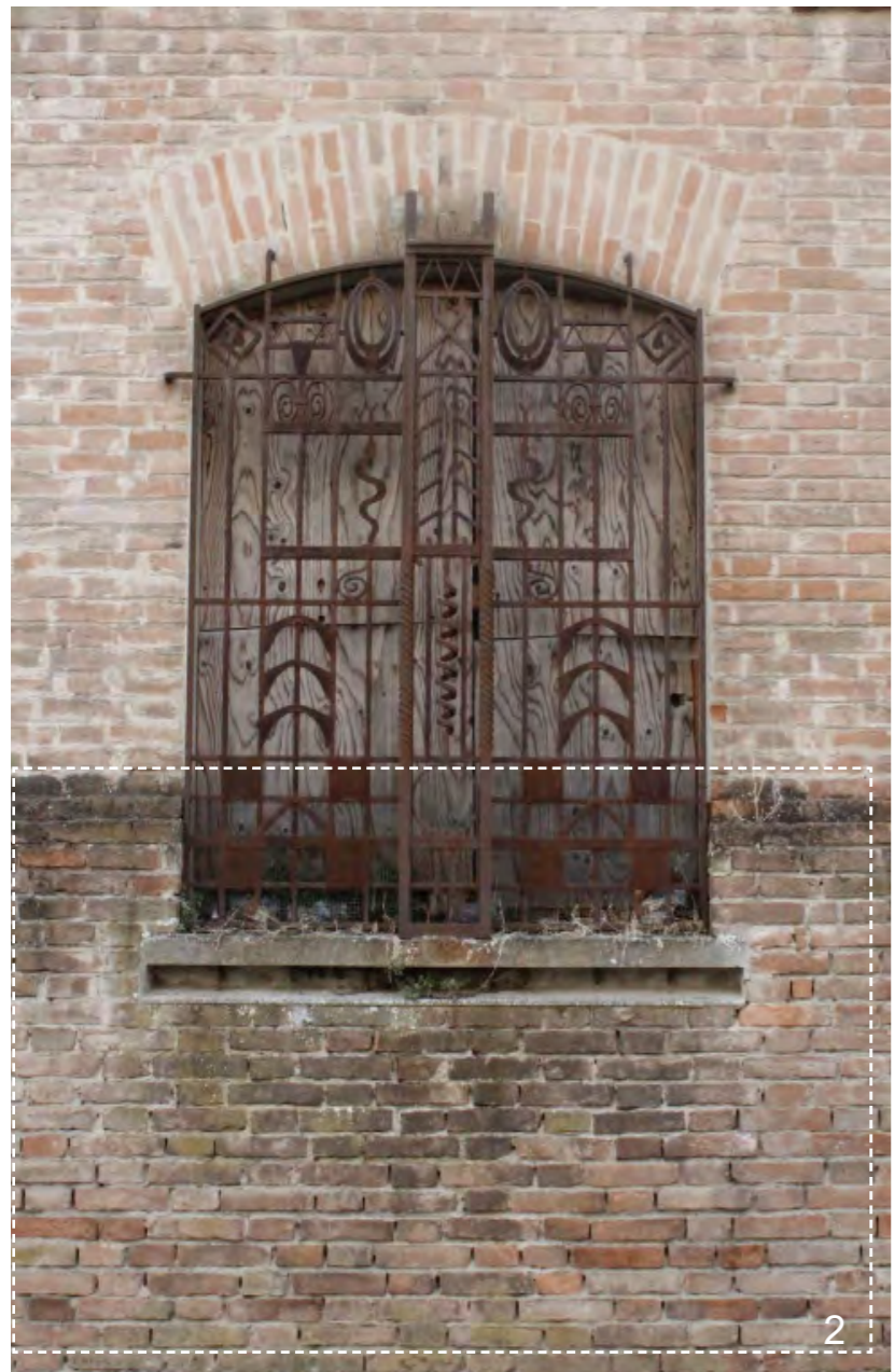
2-dripping; biological patina: the phenomenon is linked to inadequate water disposal..
