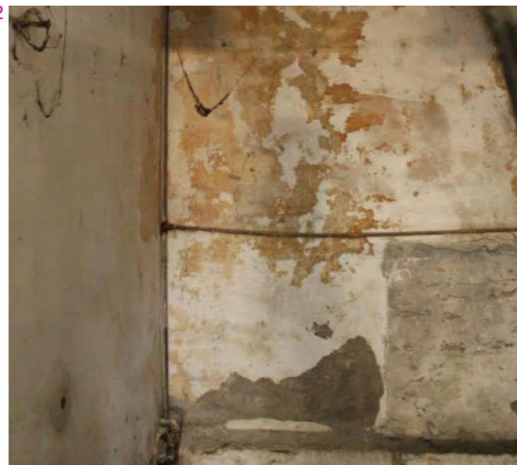
1-2 staining: a localised colour variation on the surface, related to the presence of water
