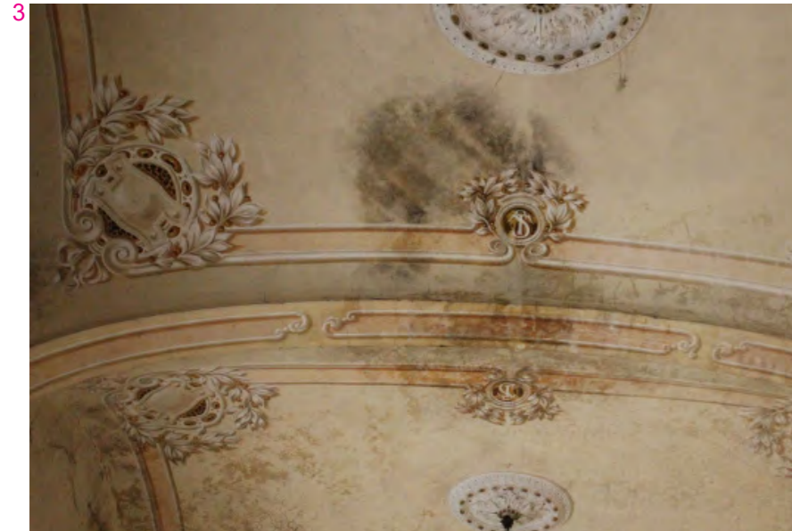
detail of the vaulted ceiling GF_0.1.002
