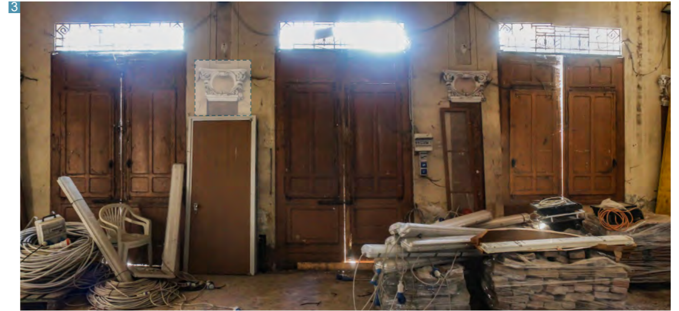
GF_0.1.002 detail architectural elements
