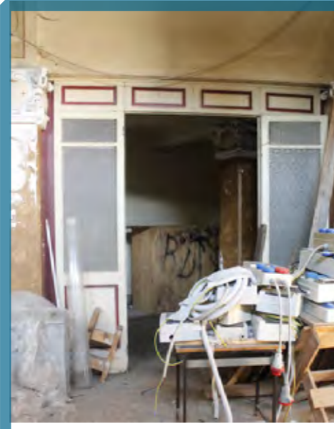
GF_0.1.002 - detail architectural elements
