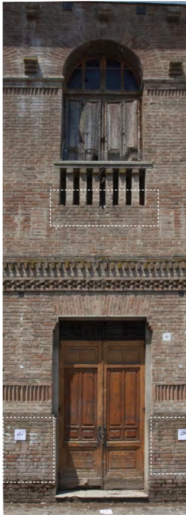
dripping; biological patina: the phenomenon is linked to inadequate water drainage, often caused by the absence of pavement markings.
