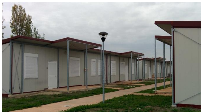
Figure 2. PMARs installed after the 2012 NIE.
