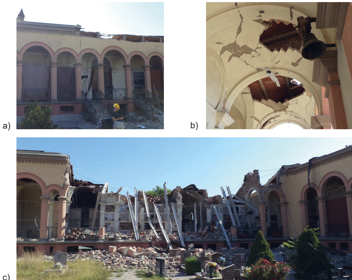
Fig.35. Cemetery of Concordia sulla Secchia: a) roof structure in reinforced hollow core slabs leaning on transversal walls; b) roof structures with reinforced concrete beams and hollow core slabs with different frameworks; c) collapse of reinforced concrete structure at transversal frame (trusting effect).
