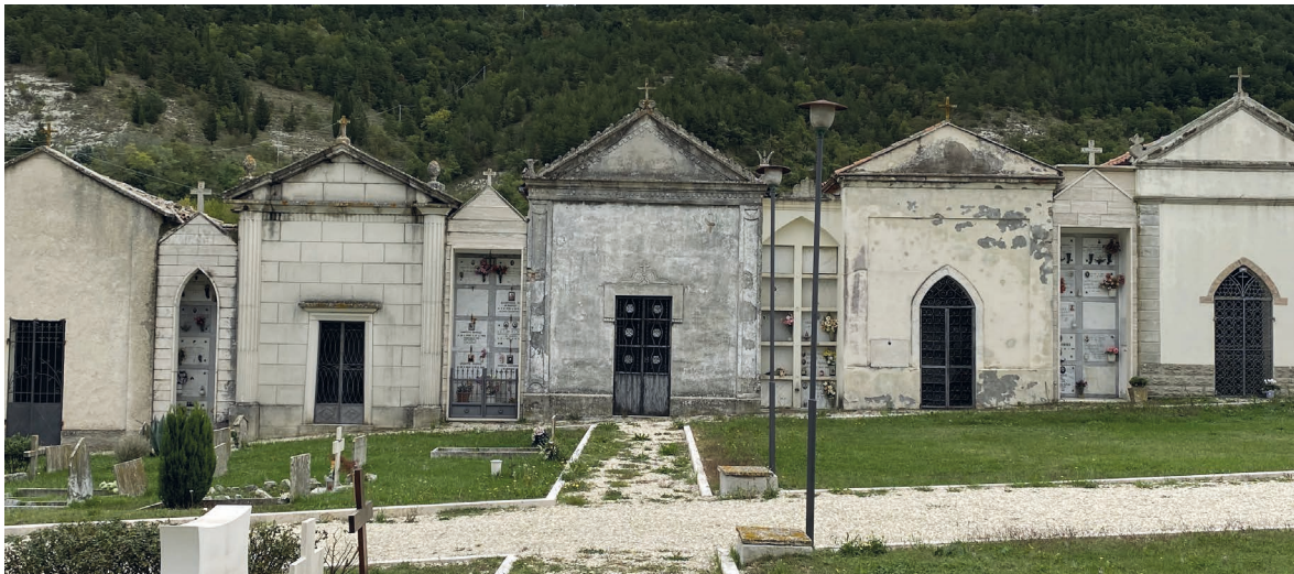
Fig.20. Cemetery of Scheggia (PG) - Centre Italy. The cemetery to overcome the problems of declivity uses the columbarium structure in the plane and an alternation of chapels and small ossuaries connected to each other for the steep parts.
