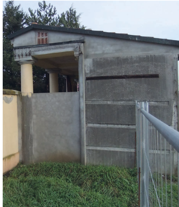
Fig.17. Migliarina Cemetery (Modena crater area). The irons of the reinforced concrete beams are left out to be used in future enlargements.
