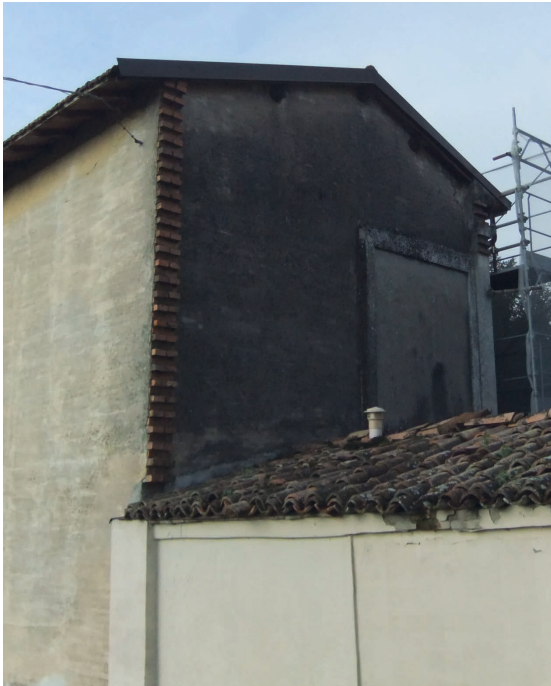
Fig.16. Budrione Cemetery (Modena crater area). Note the bricks set up for the future extension of the columbarium system.
