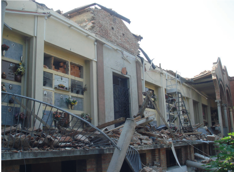
Fig.31. Cemetery of Cortile (Modena crater area), the porch in front of the columbarium collapsed.
