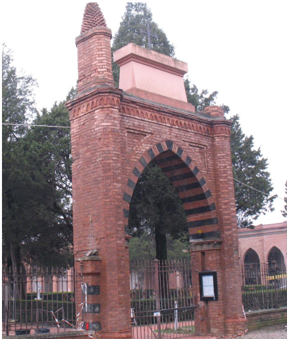
Fig.36. Cemetery of San Felice sul Panaro (Modena crater area). Collapse or damage of the projecting elements of monumental entrances
