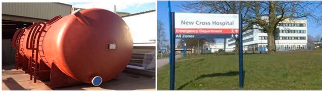
Fig. 28. Warm TES application in a UK hospital [38].
