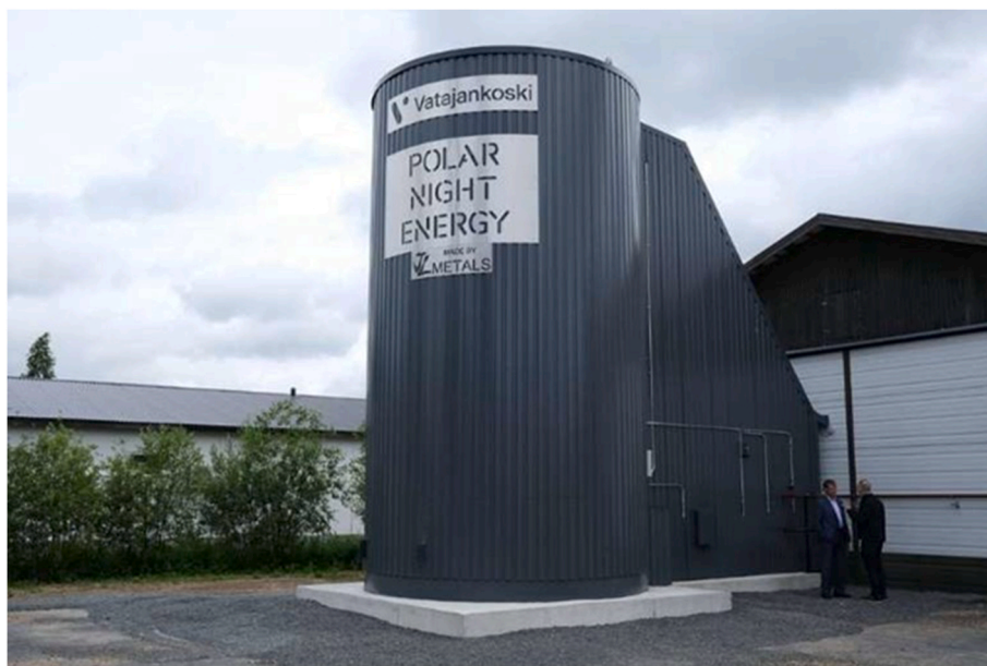
Fig. 33. Sand-based STES installation in Finland [130].
