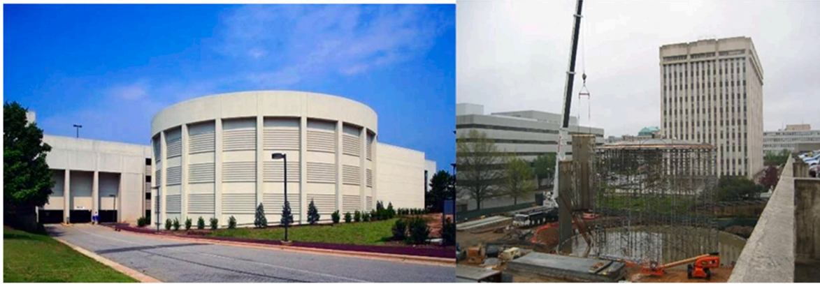
Fig. 34. Chilled water STES in the US [131].
