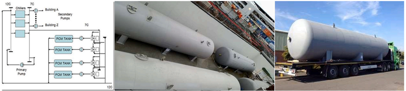
Fig. 9. Installed TES capacity 4 \times 60 \text{ m}^3 + 13 \text{ }^\circ\text{C} PCM solution providing total 10,000 kWh [38].
