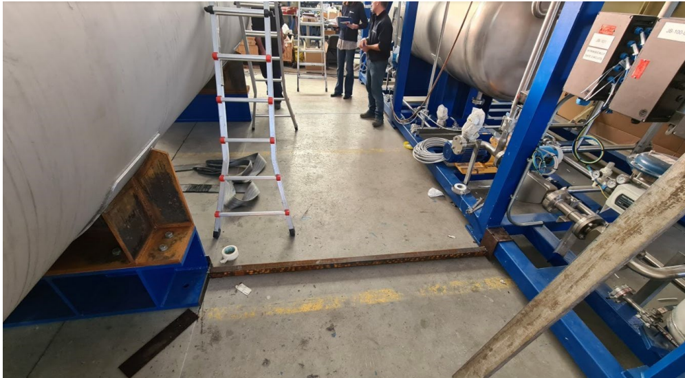
Figure 15: Metal template between T-102 tank and skid 1 for T-102 correct positioning
