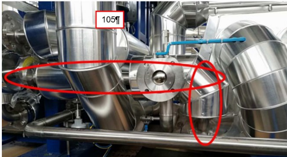
Figure 27: line 105 connecting E-104 and E-106
