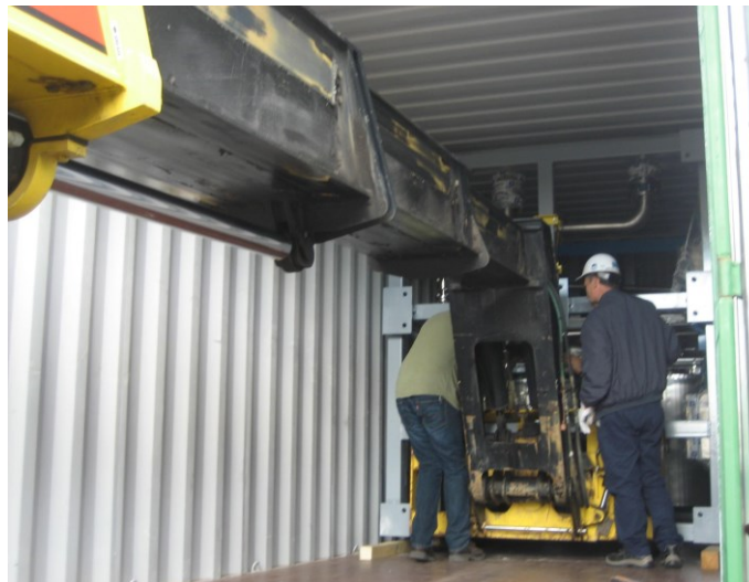
Figure 43: Connection of the forklift to the skid
