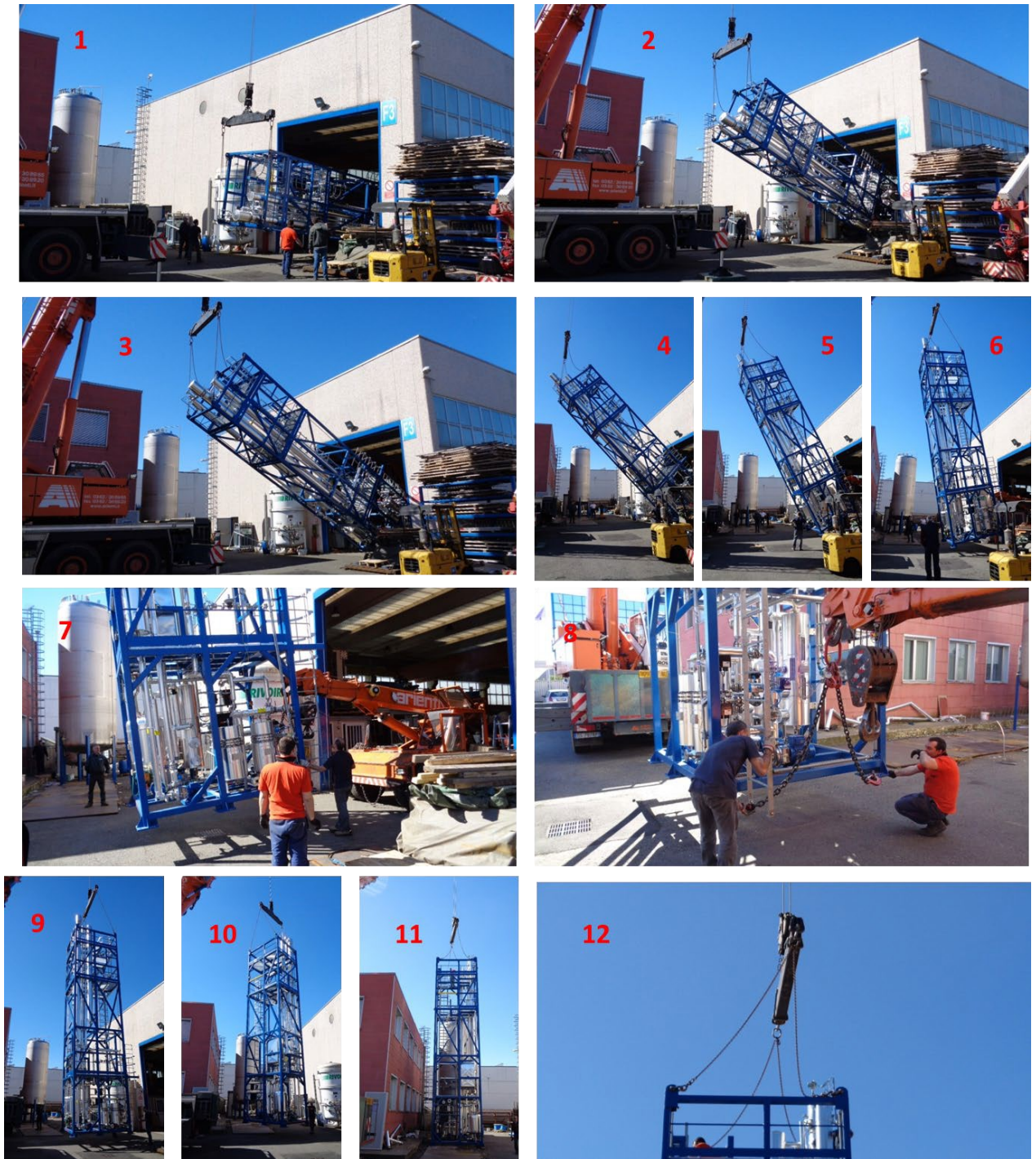
Figure 9: Erection sequence for a vertical skid
