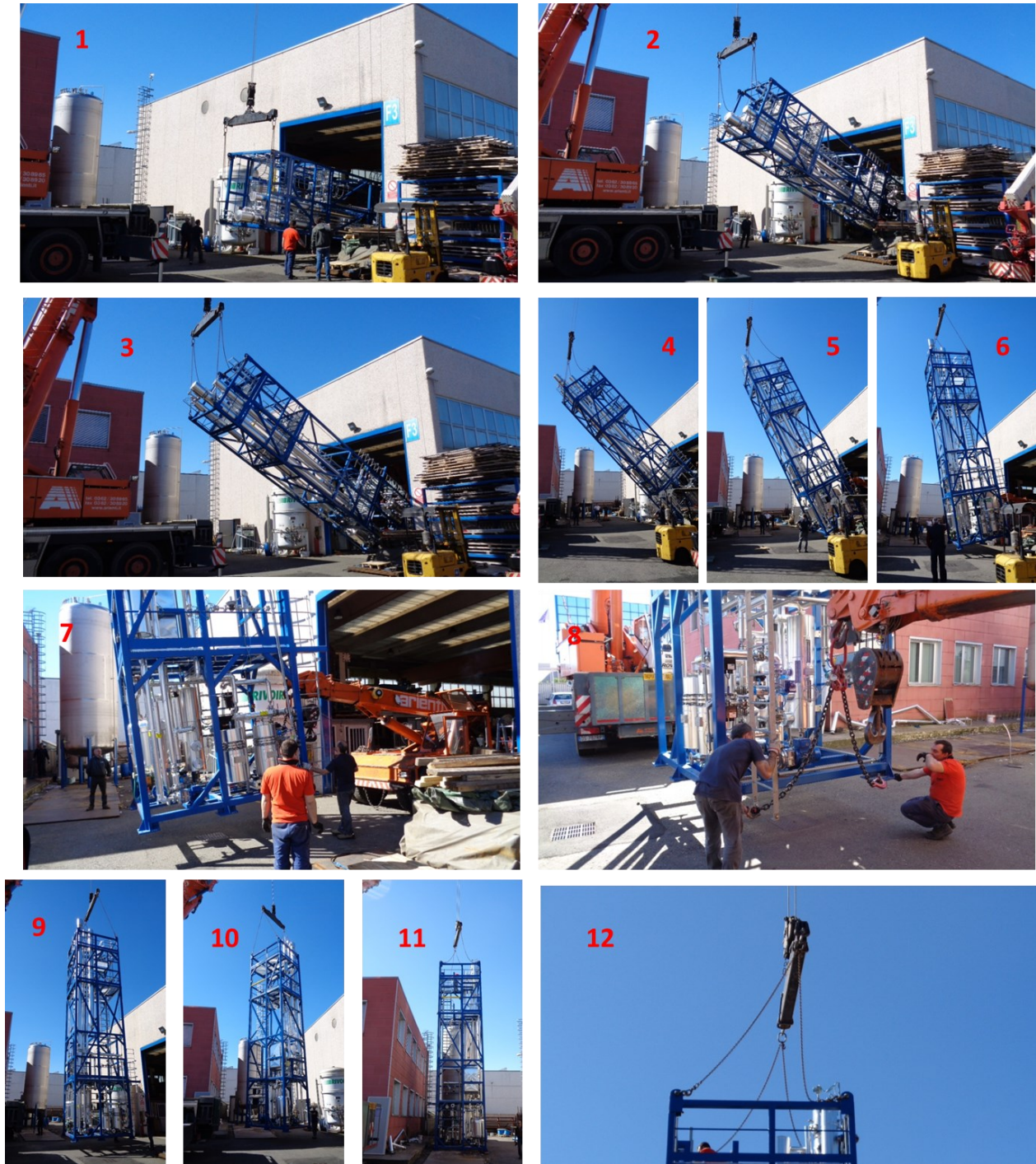
Figure 54: Skids erection sequence
