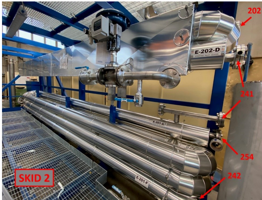
Figure 59: Blind flanges of skid 2 to be removed before the installation of skid 3 on skid 1. Leave the connection 241 and 242 with blind flanges on.
