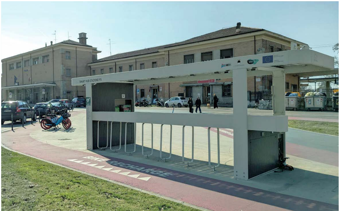
Figure 1.3. Air-Break Smart Hubs, an innovative urban services installed in Ferrara. (source: author)
