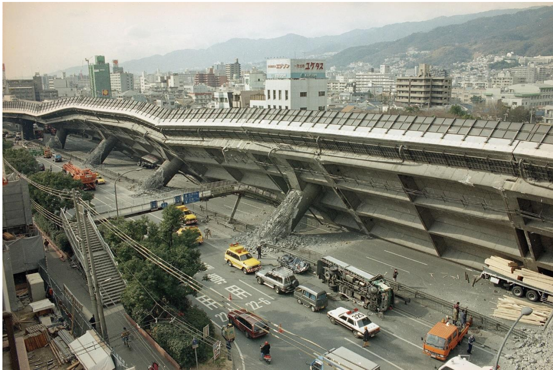
Figure 1.5 Toppling of Kobe- Osaka highway due to the Kobe Earthquake of 1995 (japantimes.co.jp)
