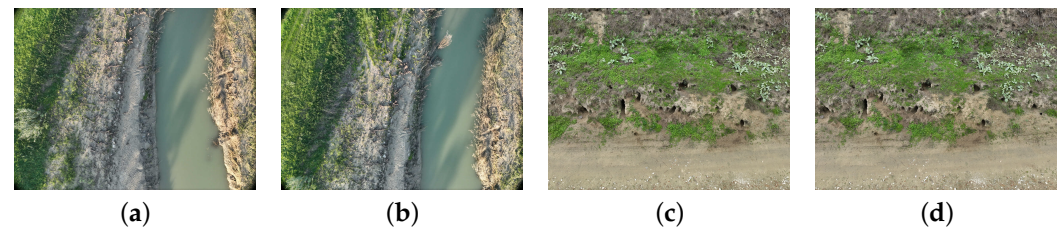
Figure 1. Examples of collected images: (a,b) show a nadir view of the river, figures (c,d) show the specific details of burrows along the levee.
