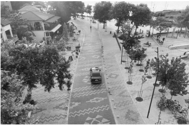
Figure 6: Shiroke, Shkoder, Albania (Albanian Carpet is a patterned plaza. Top image: it is made from blocks of granite).
