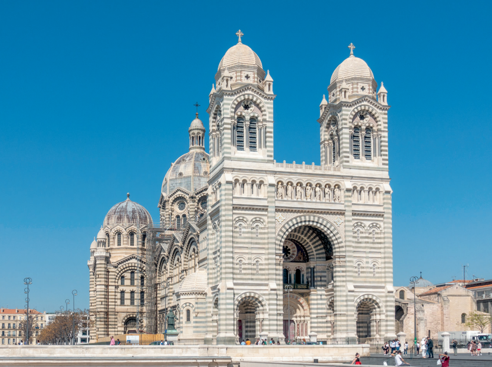
[fig. 1] Léon Vaudoyer, Henry Espérandieu, Henry Révoil, Cathedral of Sainte-Marie-Majeure, Marseille, built 1852–1893
