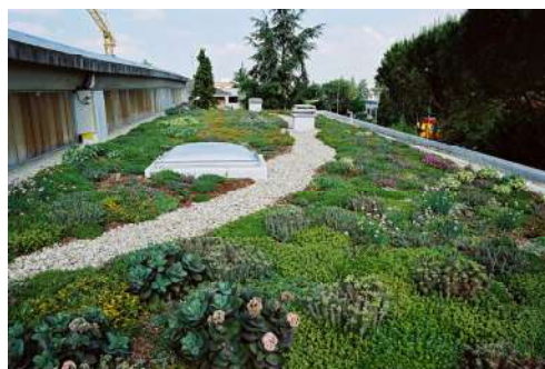
Fig. 1 – Intensive green roof, Italy
