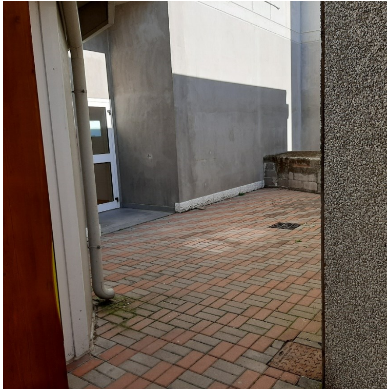
Figure 7. Space outside the dialysis centre at Cona Hospital, Ferrara.
