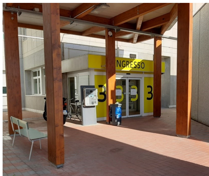
Figure 6. Space outside the dialysis centre at Cona Hospital, Ferrara.
