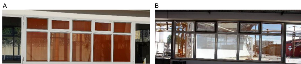
Figure 5. Pictures of the prototypes installed in the Eni Renewable Energy, Magnetic Fusion and Material Science Research Centre in Novara (Italy) viewed from the A) outside and the B) inside of the building. The Prototype 3 used for the indoor characterizations of Figure 7 corresponds the central module, whereas Sample 5 on which the in-depth analysis were performed (see Figure 8A and Table 2) is the rightmost and the leftmost device in Figure 5A,B, respectively.
