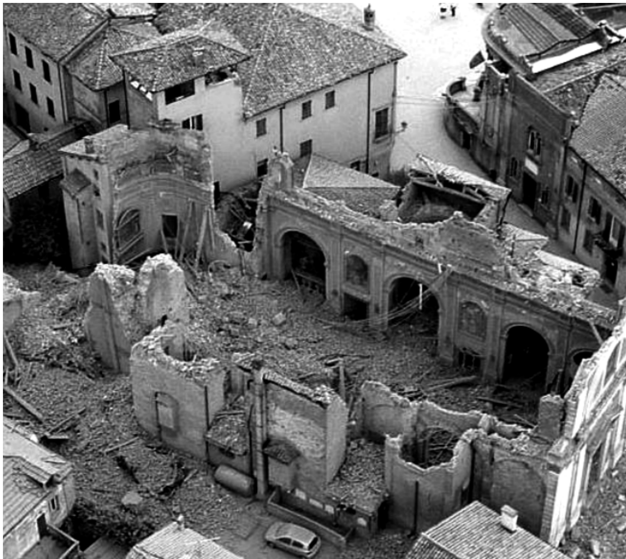
Fig.15 - Damage caused by the 2012 earthquake - ARREER photo archives.
