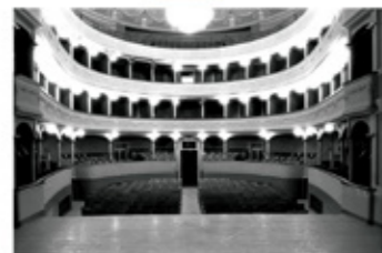
San Felice sul Panaro, Teatro Comunale, the hall before the restoration (photo Riccardo Vlahov, IBC) 1980, 20334001
