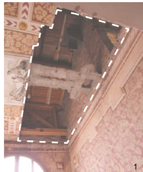
LOCAL COLLAPSE OF CEILING OR VAULT - M16
