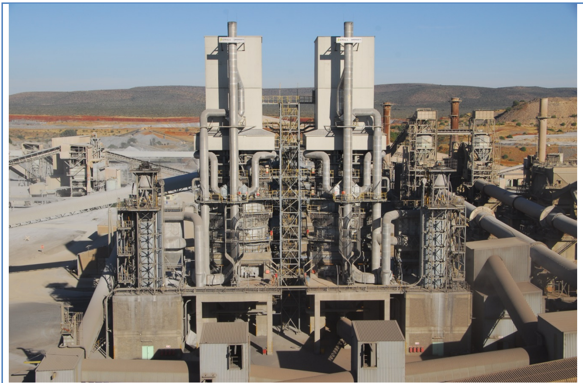
Fig.3.10: Panoramic view of TSR Kilns 9 and 10 installed at Idwala Plant by Cimprogetti in 2013-2014.
