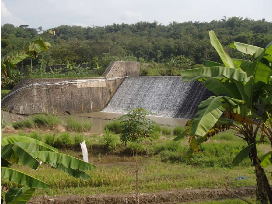
Figure 27. Cemoro dam at the Sangiran dome
