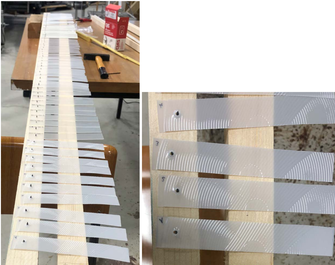
Figure 21: a) Assembly phase of the plastic strips on the wooden slats. b) Detail.
