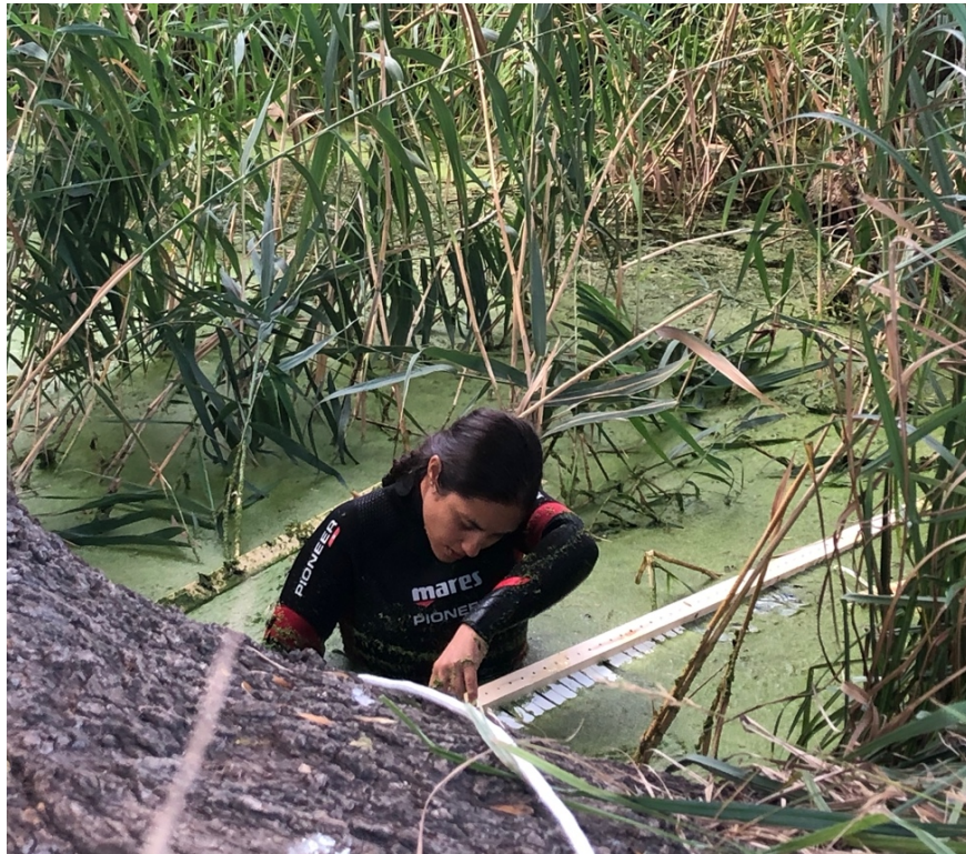
Figure 29: Installation of the slats in the Ciane river in semi-floating condition.
