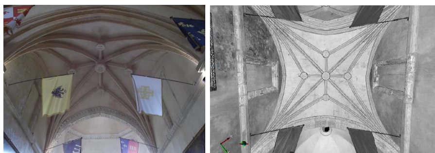
(a) Stellar vault located at the presbytery (b) Geometric outline of the vault obtained by laser scanning techniques
