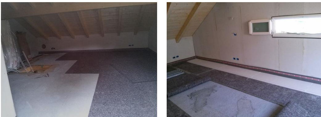
Figure 17 – second floating floor realization
